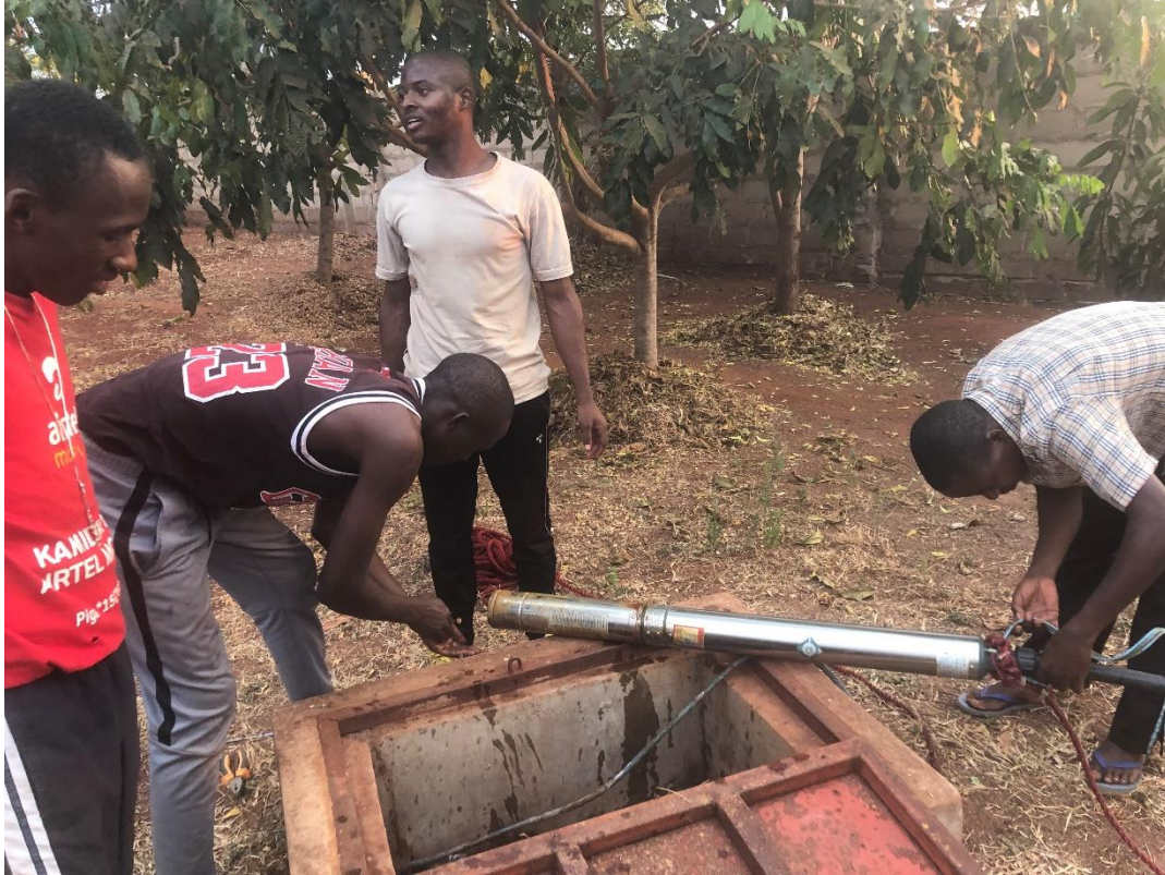
Francis, Gervas, Peter and Phillip did most of the “hands on” work. I was standing ready with advice. Below, “we” are putting the pump back into the well with the 80 meter hose.
