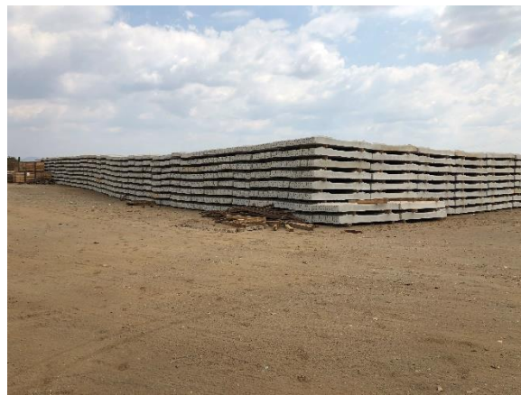
Concrete slabs stockpiled to be used as foundations for the rails.
